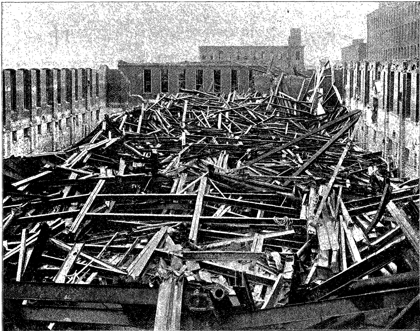
The St. Louis storm, 1896. This was the scene of several deaths. The building in course of construction was part of what was designed to be the largest tobacco factory in the world, at an expenditure of $1,500,000. The workmen sought refuge in the cellar, but the steel framework fell through on them, and but few escaped with their lives.
